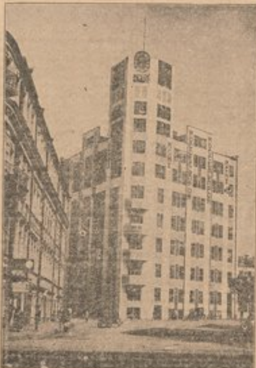
"Moselproom," one of the many spa class, sanitary and therefore, healthful factories of the Soviet Union. It is building is located in the heart of the city of Moscow. Note the many windows that shed light in every part of the building and compare it to the sordid, dark, miserable factories where workers slave from eight to twelve hours a day in the United States. All workers in the former factory pictured above work seven hours a day, and a five-day week. The factory above makes cigarettes and confectionary.
