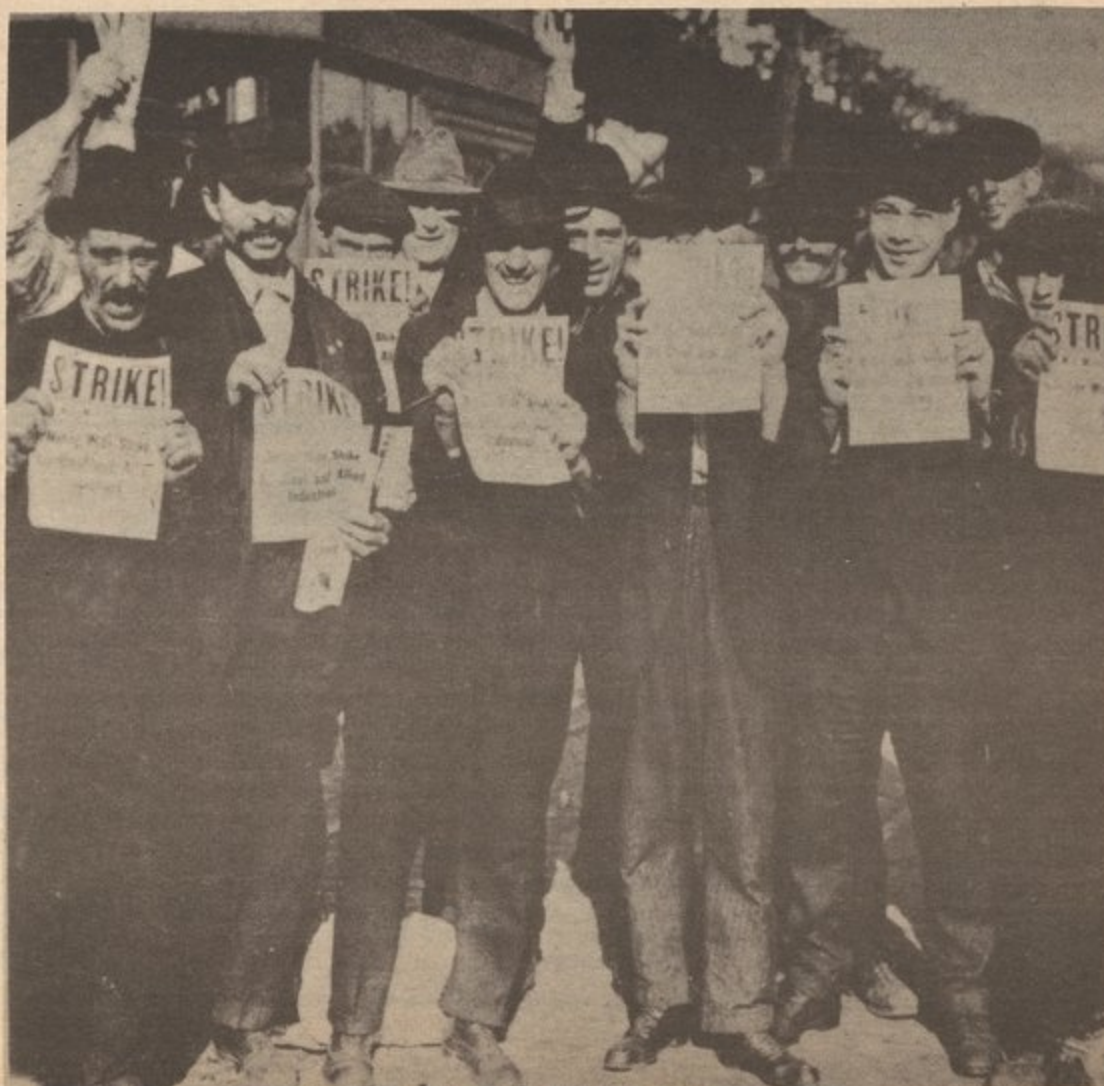
Chicago steel workers, 1919.
