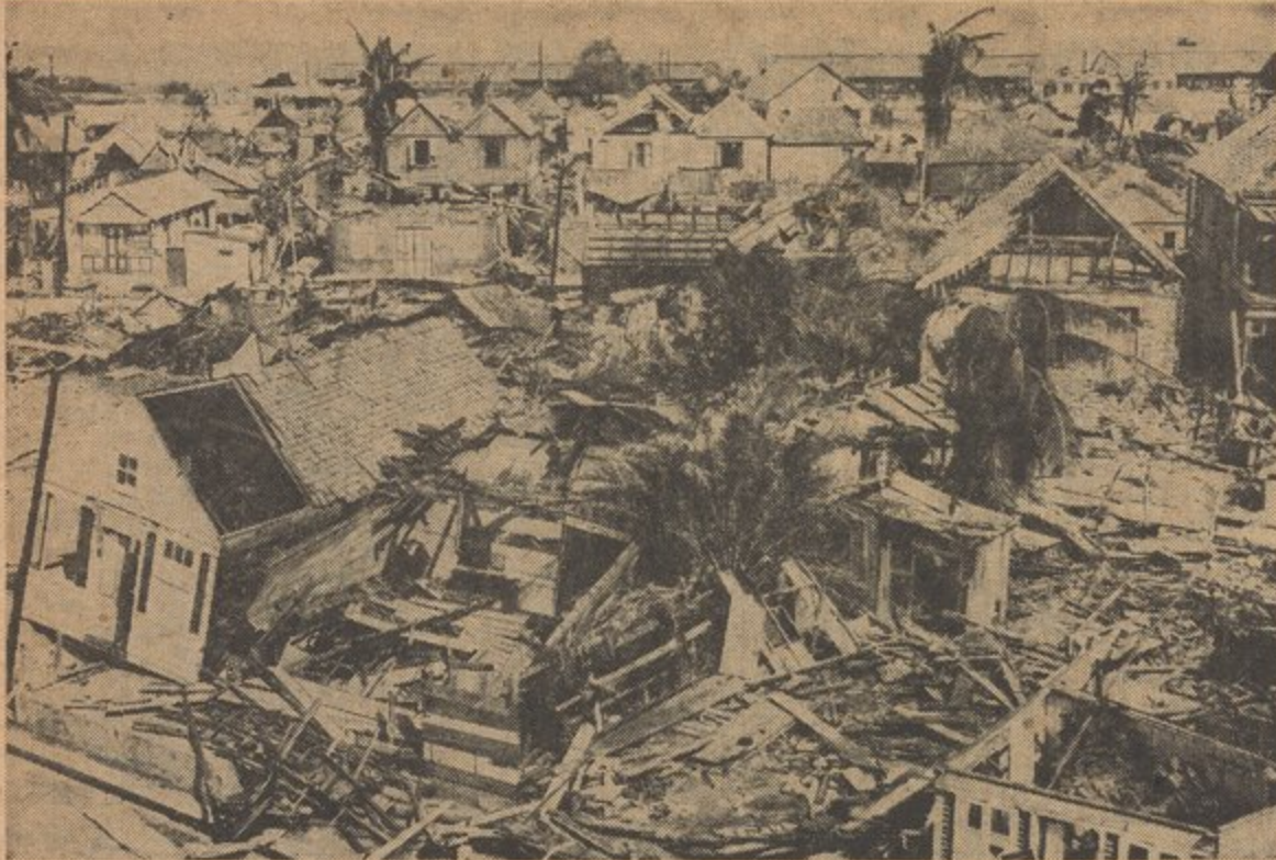
JAMAICAN FISHING VILLAGE of Port Royal lies nearly flat after the hurricane blasted it. Hardly a house was left intact. Money, food and clothing are desperately needed for the thousands of homeless all over the island.
