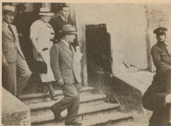
Chile's Popular Front president, Aguirre Cerda, inspects the earthquake-stricken town of Talca
