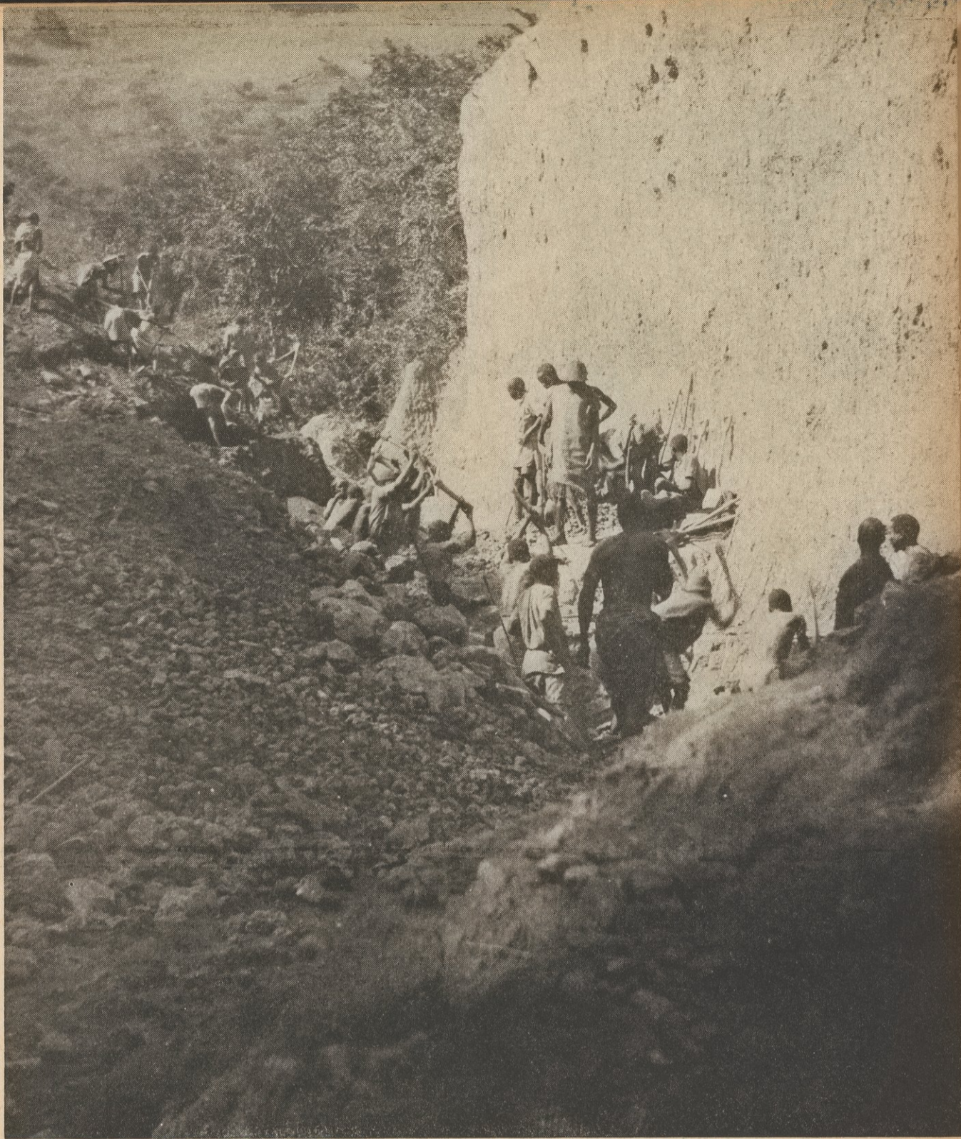
Excavating for alluvial tin in a creek in Tanganyika
