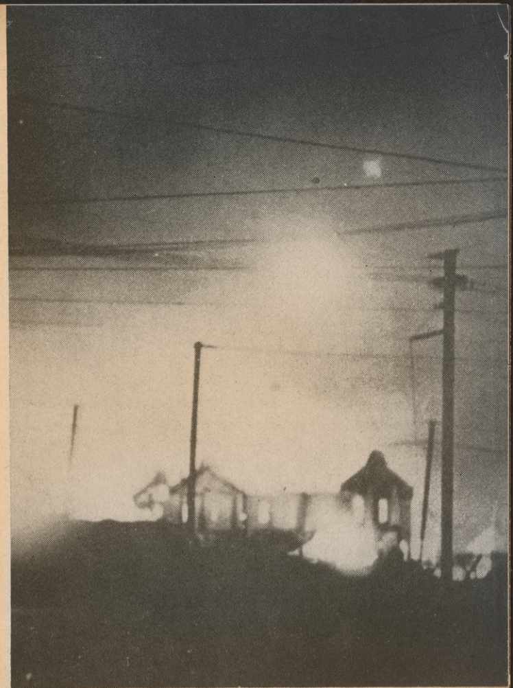
Chapei—"saved at last"
