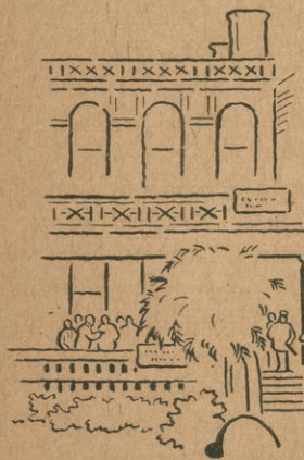
Machinists' Hall, 113 S. Ashland Boulevard.
