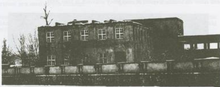
Fig. 5. Kabul National Museum showing replacement windows, Afghanistan
