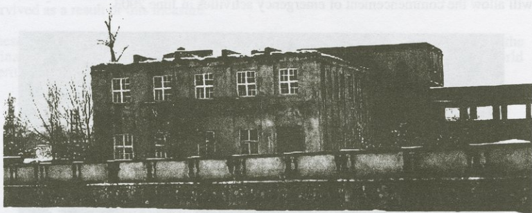
Fig. 5. Kabul National Museum showing replacement windows, Afghanistan
