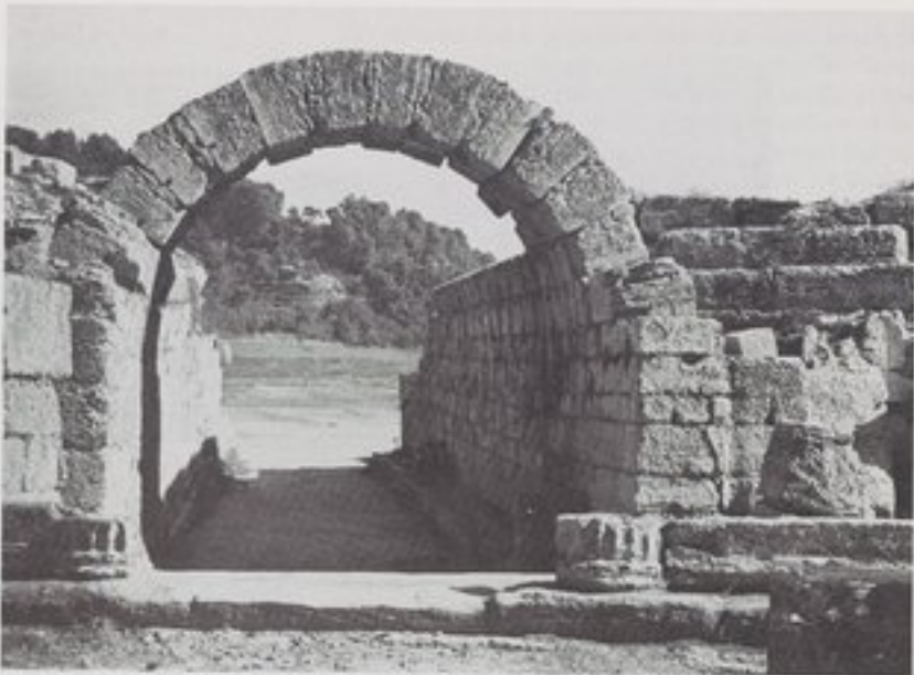
5. Olympia Stadium vaulted entrance, as seen from the west. A portion of the vault has been reconstructed in the modern day. Photo DAI, Athens, neg. nr 72/3967.
