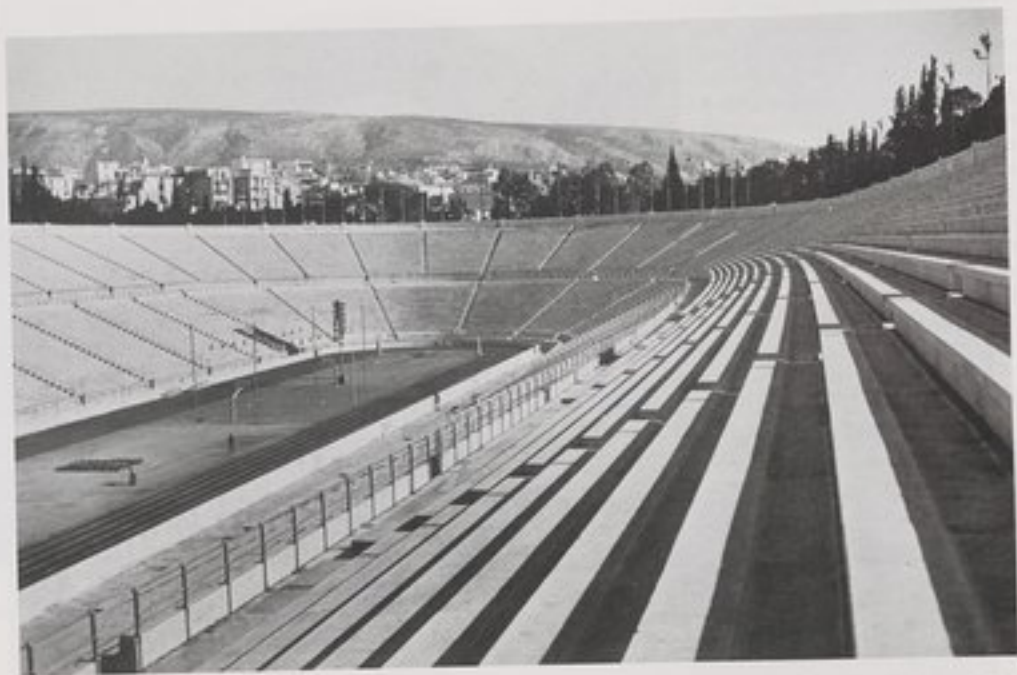
6. The Panathenaic Stadium in Athens, originally built in the second century A.D. and reconstructed for the first celebration of the Modern Olympic Games in 1896. Photo by the author.
