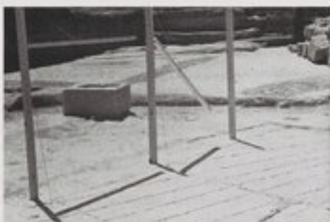
43a. Isthmia, Photograph of the bullhides sill with restored wooden gates. Photos courtesy of the University of Chicago, Isthmia Excavations.
