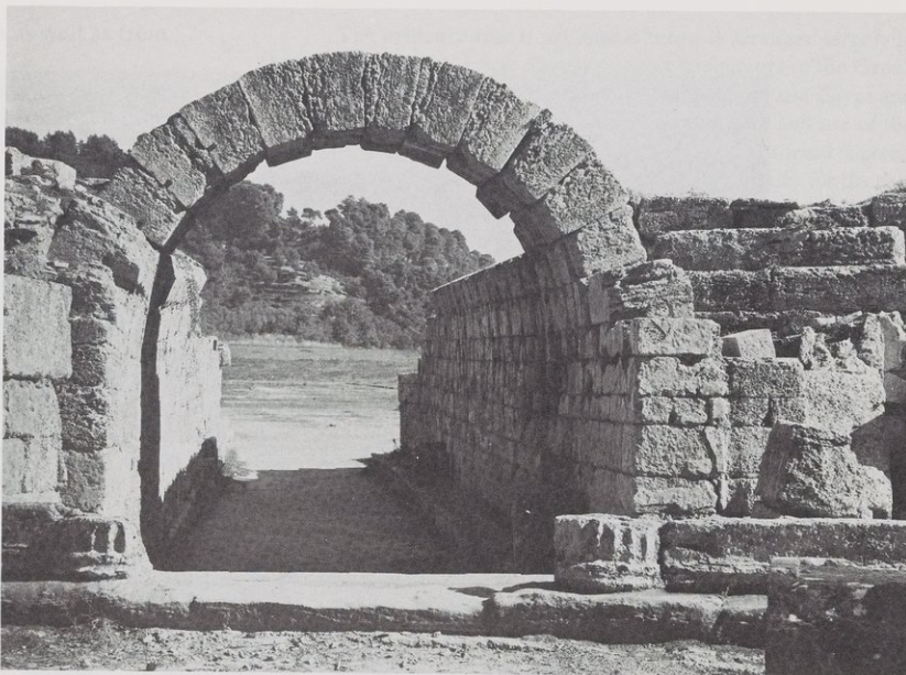
5. Olympia Stadium vaulted entrance, as seen from the west. A portion of the vault has been reconstructed in the modern day. Photo DAI, Athens, neg. nr 72/3867.
