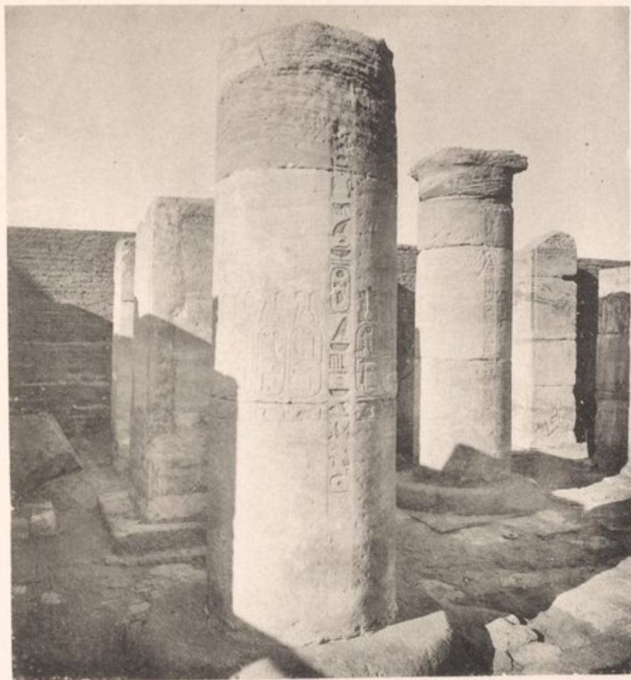
a. Columns in southern half of forecourt.
