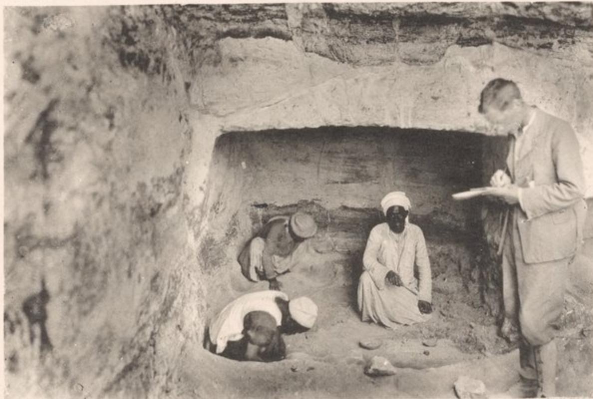
K 32. The process of excavating and noting.
