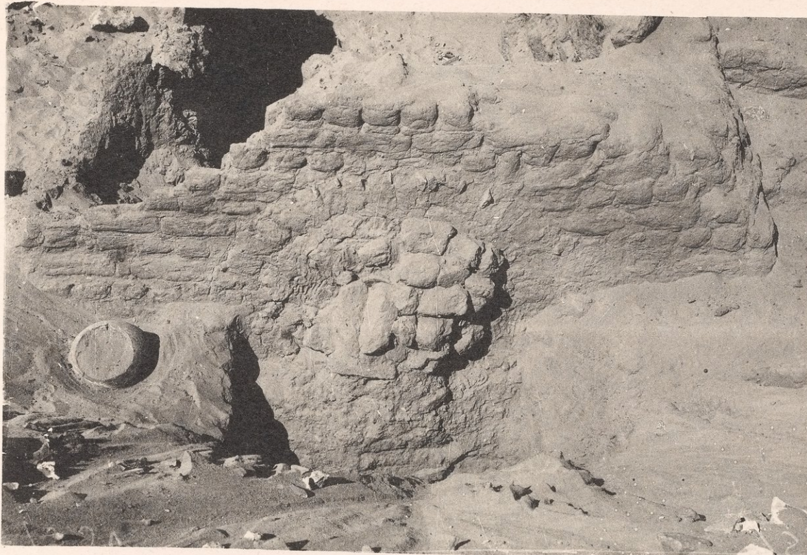
K 44. Brickwork of the east end, outside.
