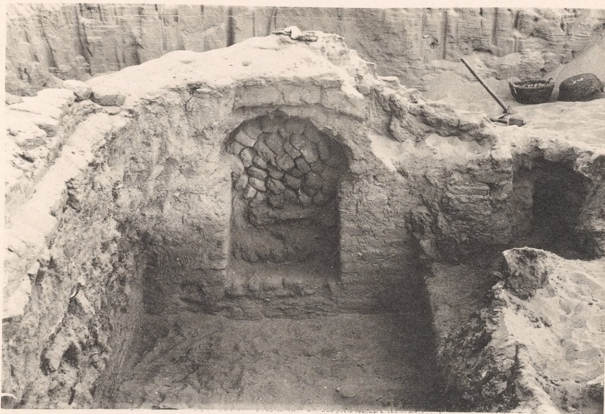
K 44. Brickwork of the east end, inside.
