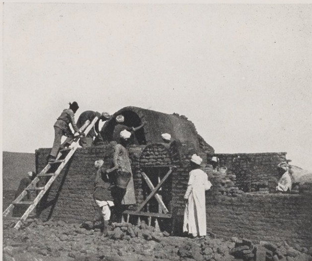
Modern Nubians building arch and barrel vault; Wady Halfa, 1909
