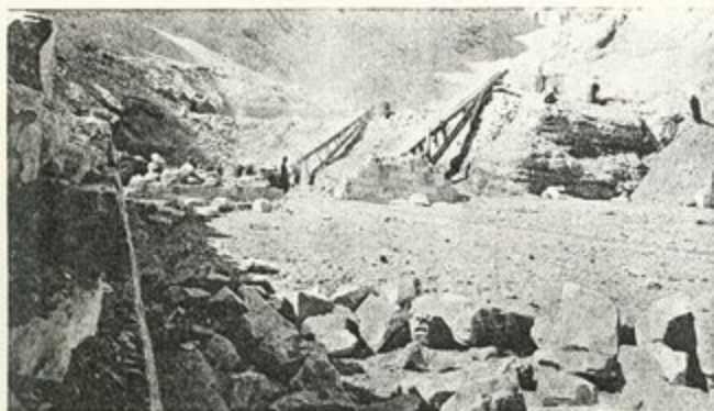
1. CLEARING THE TEMPLE PLATFORM: THE SHOOTS AT WORK IN THE SOUTHERN COURT
