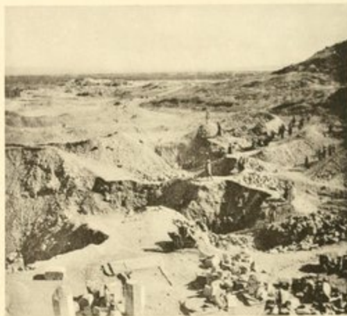
Digging the Great Trench, Nov. 1904.
