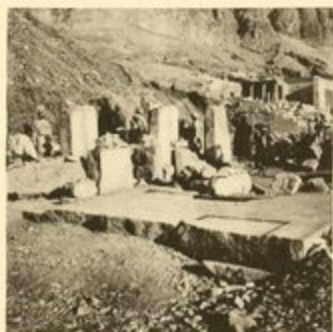
Excavating the Platform, Jan. 1904.
