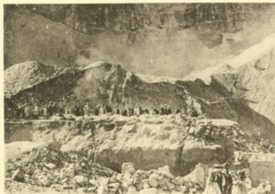
The Excavation, Dec. 1903.
