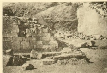
The North Cross-wall and Court.
