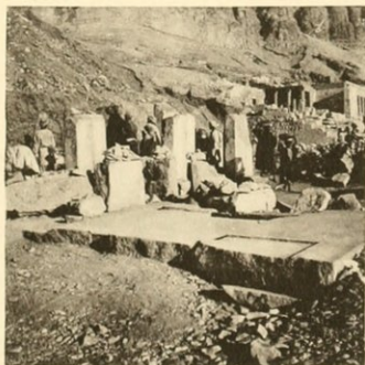
Excavating the Platform, Jan. 1904.
