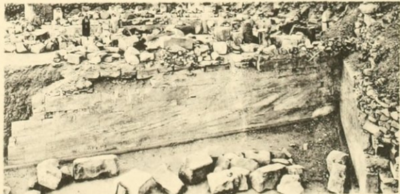
North lower court showing sharp angle of walls. Borchardt
