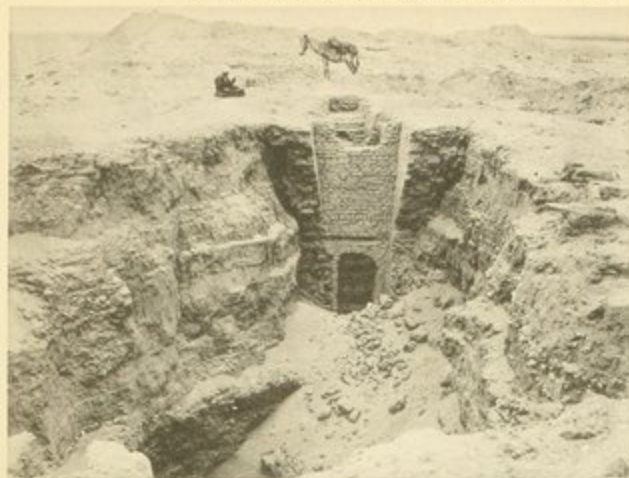
SUB-STRUCTURE AFTER COLLAPSE
