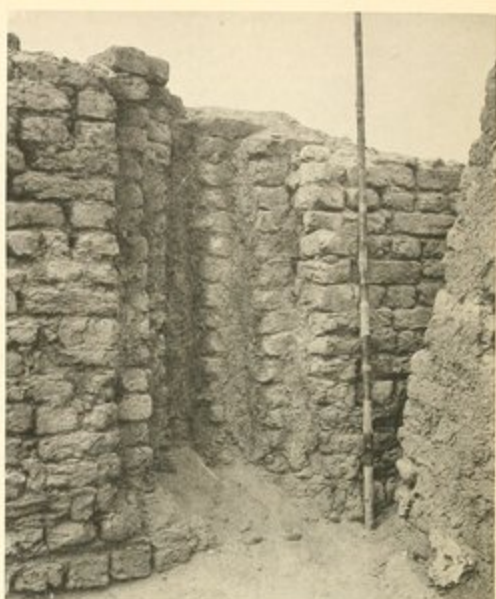
PANEL RECESS, EAST WALL
