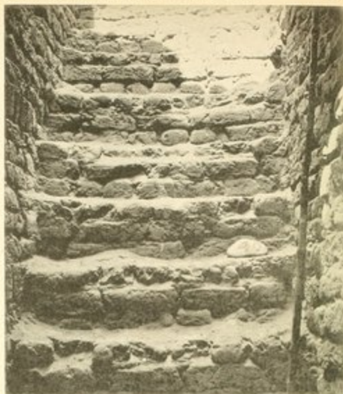
STAIRWAY DESCENDING IN BRICK STEPS.
