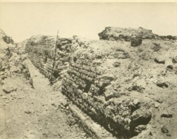
WEST WALL, FROM S.
