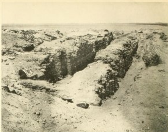
VIEW SHOWING FIRST INNER PASSAGE, FROM S.
