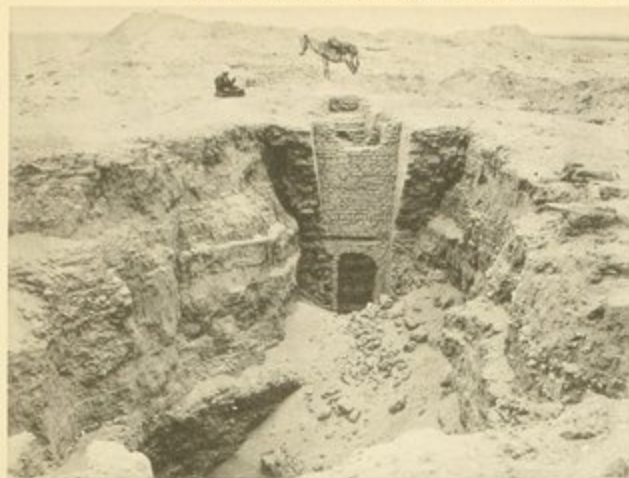
SUB-STRUCTURE AFTER COLLAPSE
