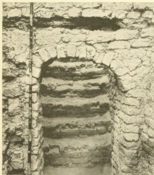
ARCHWAY AND STEPS. FROM S
