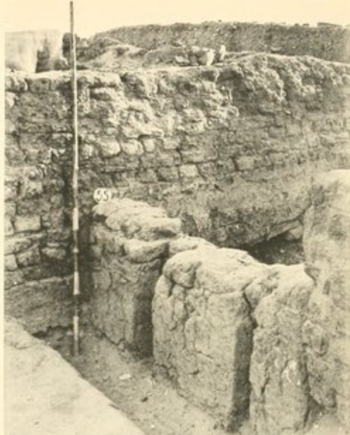
EAST FACE OF R 55a
