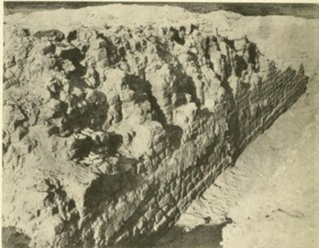
S. WALL, PARTLY PANELLED.
