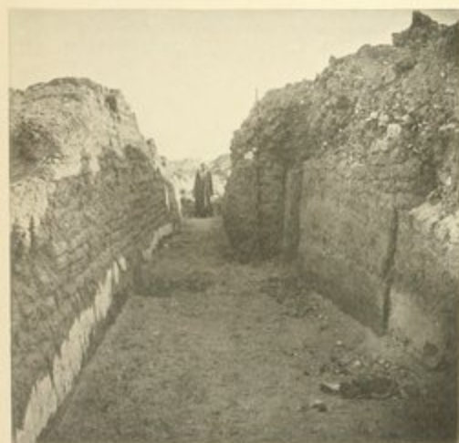
W. WALL, TO LEFT, STUCCOED.
