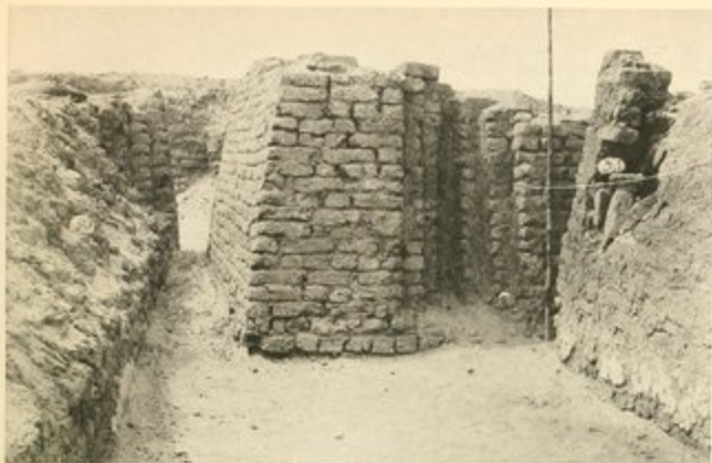
SITUATION OF TOMB STRUCTURE
