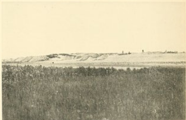
NORTHERN MOUND DURING EXCAVATION.
