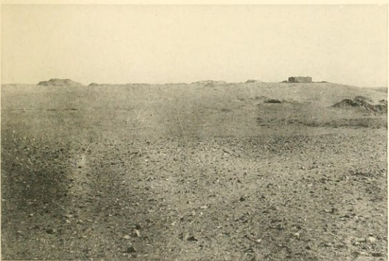
NORTHERN MOUND AFTER EXCAVATION.
