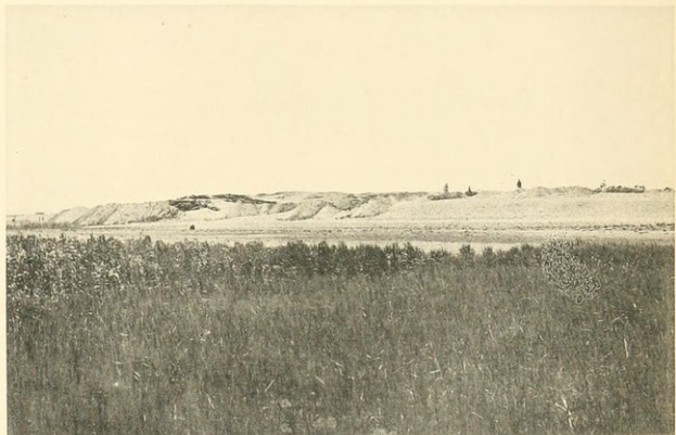
NORTHERN MOUND DURING EXCAVATION.
