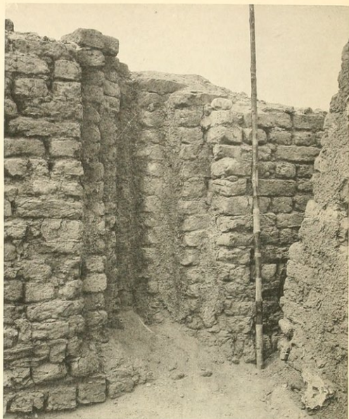
PANEL RECESS, EAST WALL
