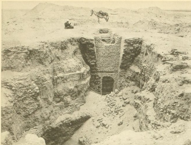
SUB-STRUCTURE AFTER COLLAPSE
