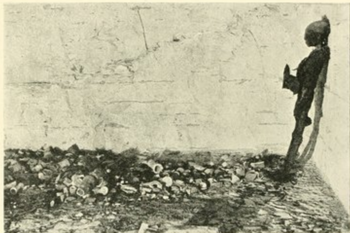
FIG. 3. INTERIOR OF SIDE CHAMBER D.
