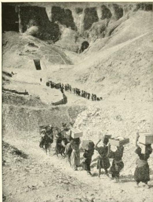
FIG. 1. PROCESSION OF WORKMEN REMOVING THE ANTIQUITIES AFTER THE OPENING OF THE TOMB.
