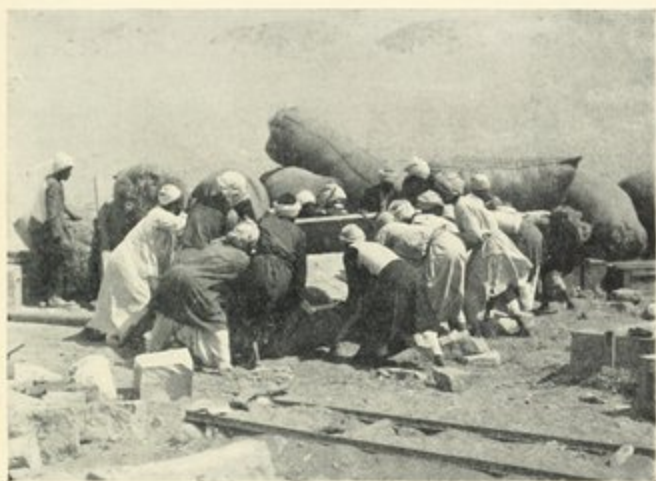
FIG. 18. PACKING LINTEL OF MAIN DOORWAY
