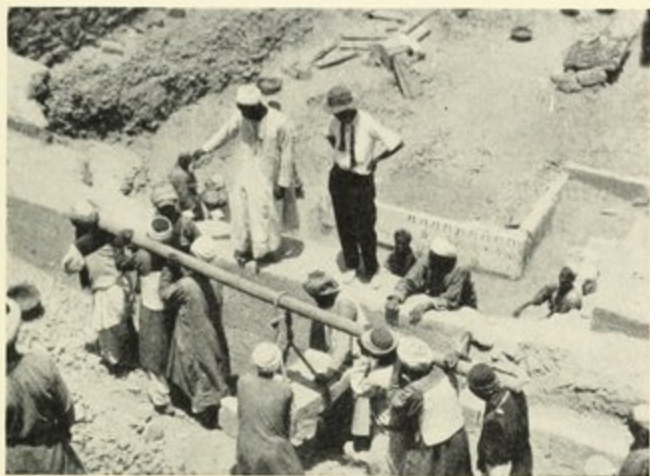
FIG. 23. METHOD OF CARRYING BLOCKS
