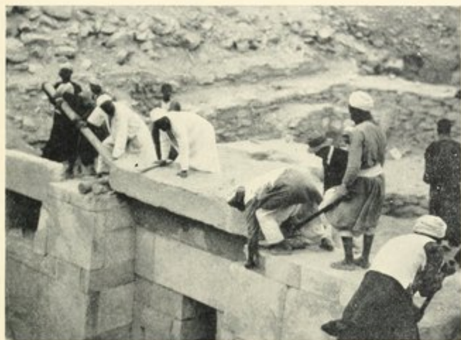
FIG. 16. REMOVING LINTEL OF MAIN DOORWAY
