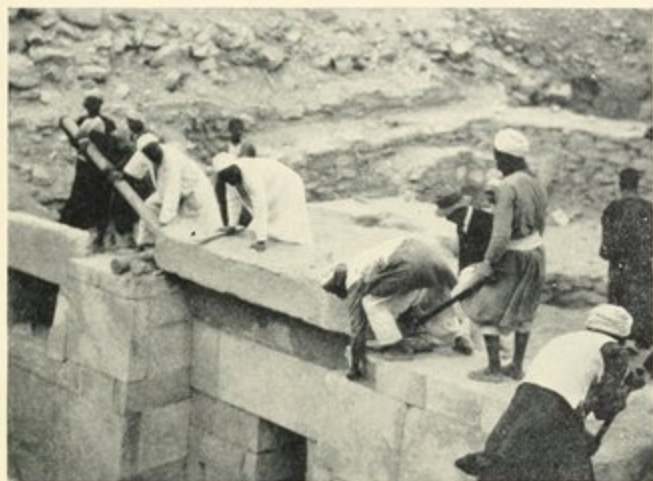
FIG. 16. REMOVING LINTEL OF MAIN DOORWAY
