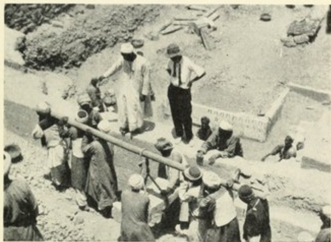
FIG. 23. METHOD OF CARRYING BLOCKS
