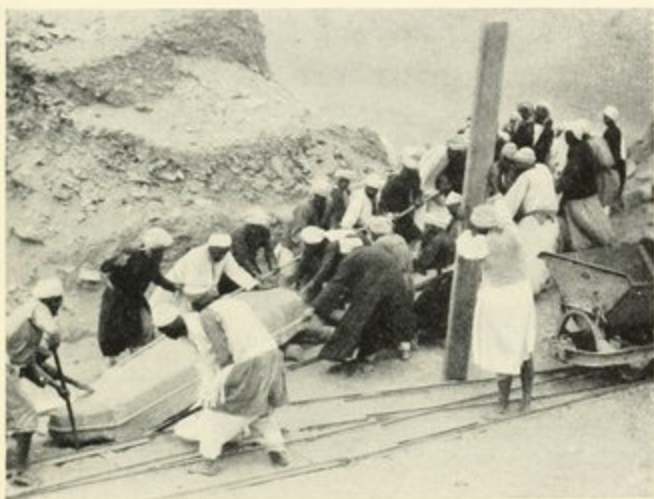
FIG. 17. HAULING LINTEL OF MAIN DOORWAY
