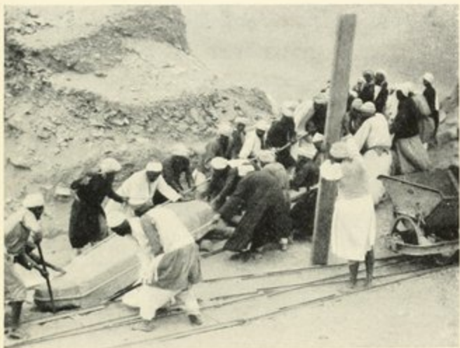
FIG. 17. HAULING LINTEL OF MAIN DOORWAY
