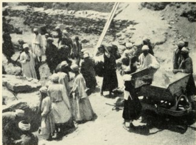
FIG. 14. PROGRESS OF THE EXCAVATIONS
