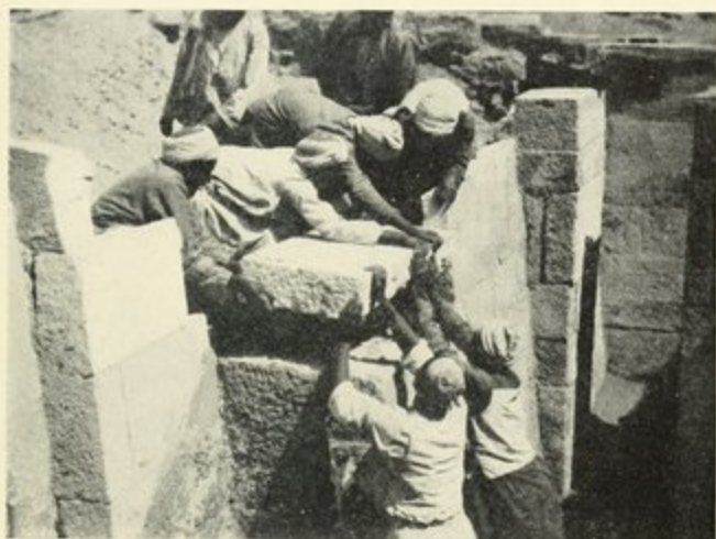
FIG. 20. REMOVING BLOCKS FROM FAÇADE
