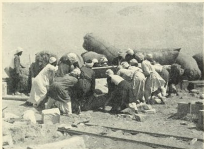
FIG. 18. PACKING LINTEL OF MAIN DOORWAY
