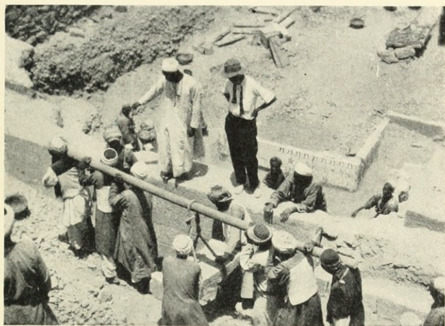
FIG. 23. METHOD OF CARRYING BLOCKS
