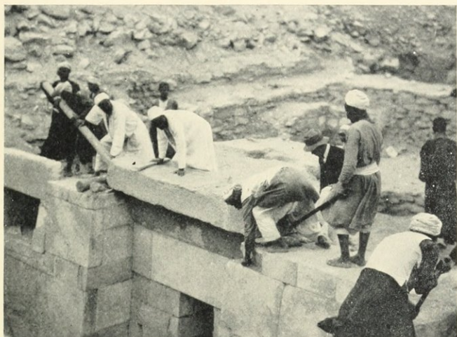
FIG. 16. REMOVING LINTEL OF MAIN DOORWAY
