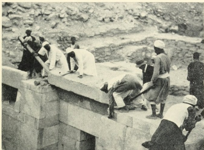
FIG. 16. REMOVING LINTEL OF MAIN DOORWAY
