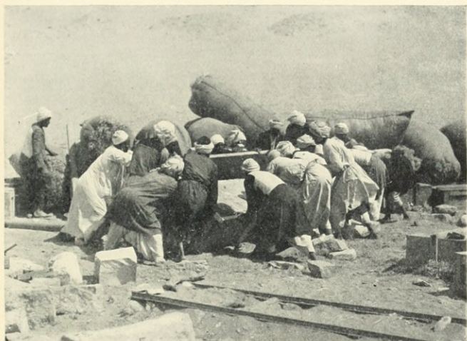
FIG. 18. PACKING LINTEL OF MAIN DOORWAY
