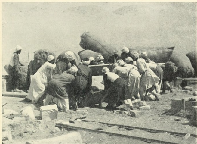
FIG. 18. PACKING LINTEL OF MAIN DOORWAY
