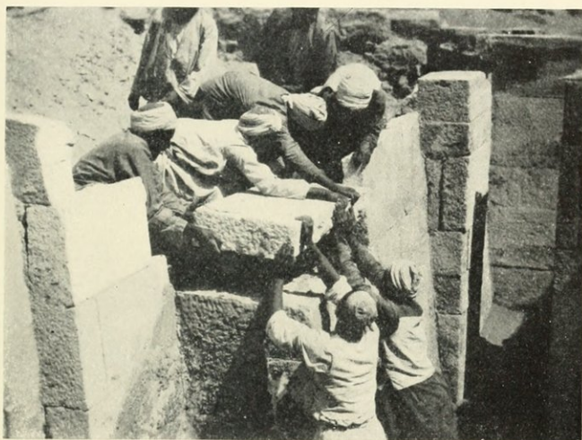
FIG. 20. REMOVING BLOCKS FROM FAÇADE
