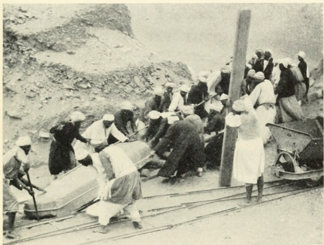
FIG. 17. HAULING LINTEL OF MAIN DOORWAY
