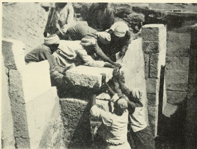
FIG. 20. REMOVING BLOCKS FROM FAÇADE
