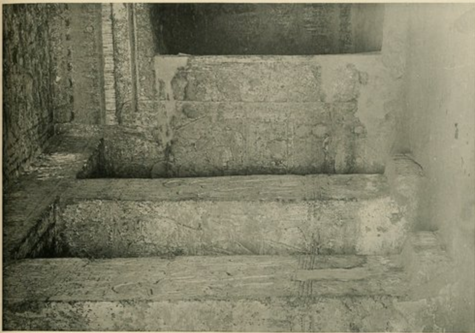
View of Second Pillared Hall looking east.
