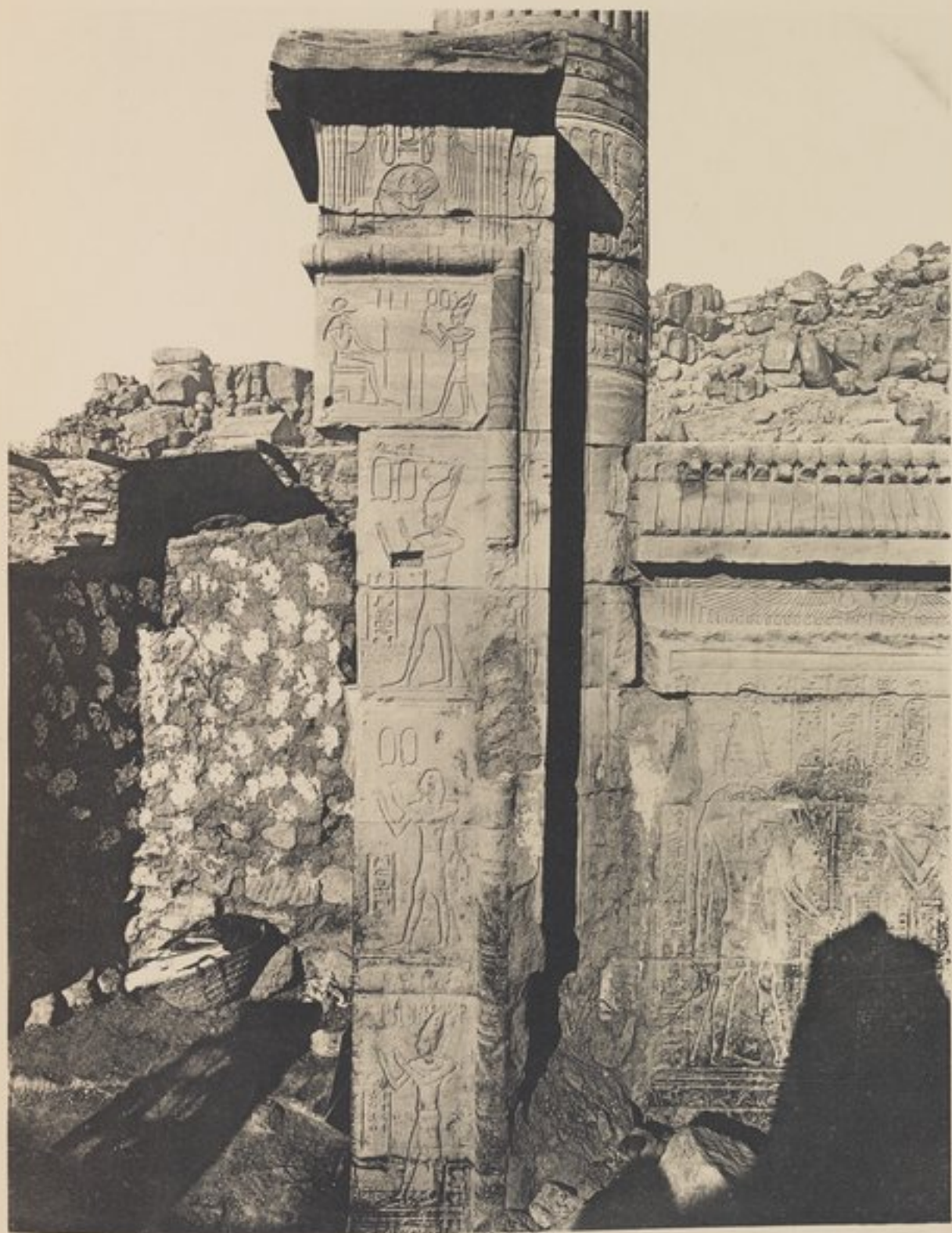
Outer Hall : Entrance : East Face : North Jamb.
