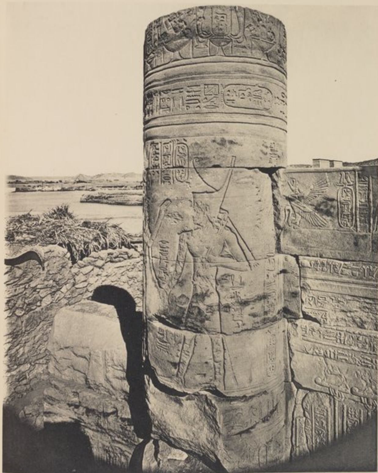
Outer Hall : West Side of Column 1.
