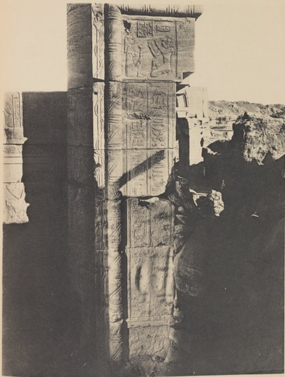
Outer Hall : Entrance : West Face : North Jamb.
