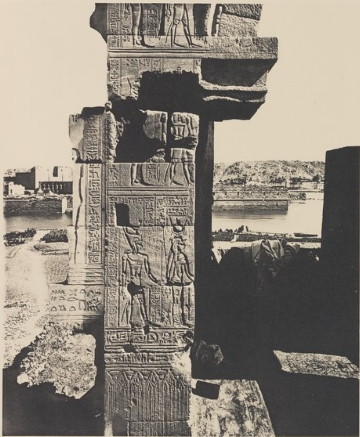
Gate-Way of Pylon : West Face : North Jamb : Scenes III and IV.
