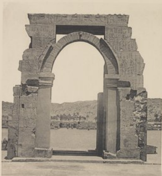
2. Gate-Way of Pylon : West Face.
