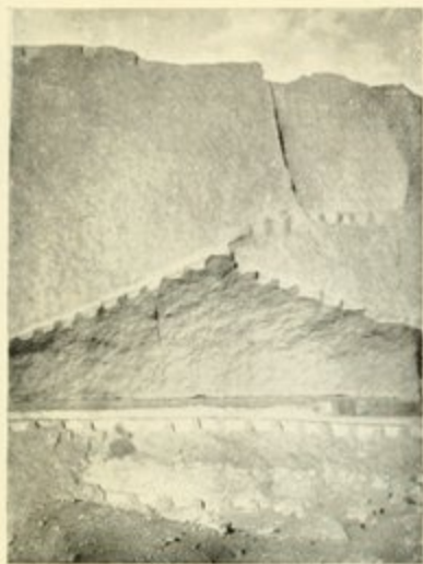
FIG. 8.—WEDGE AND CHISEL MARKS NEAR ASWAN OBELISK.
