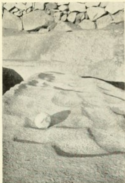
FIG. 5.—HAMMER-DRESSING ON PYRAMIDION OF ASWAN OBELISK. (Page 36.)
