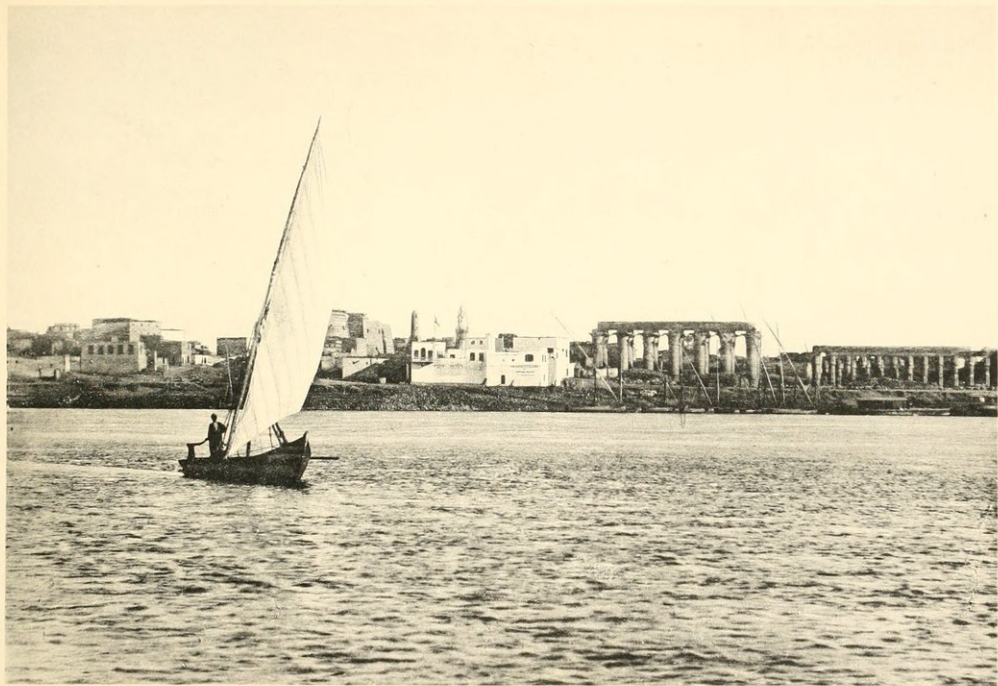
Vue générale de Luxor. — General view of Luxor.
