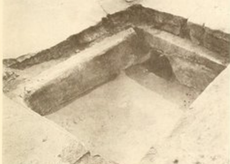
LEAD TANK OF DRAIN
