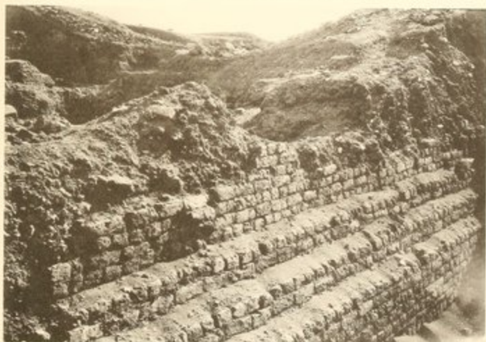
BLOCKING OF OLD ENTRANCE IN FOSSE.
