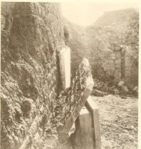
STONE LINING PARTLY FALLEN FORWARD.
