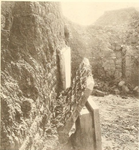
STONE LINING PARTLY FALLEN FORWARD.
