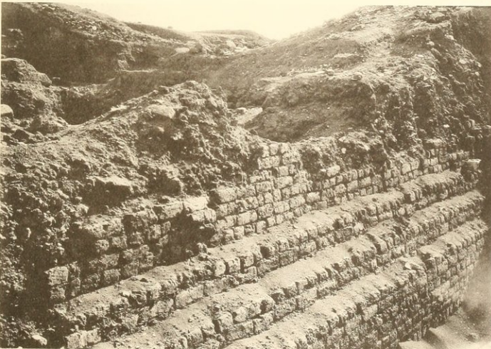
BLOCKING OF OLD ENTRANCE IN FOSSE.
