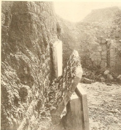
STONE LINING PARTLY FALLEN FORWARD.
