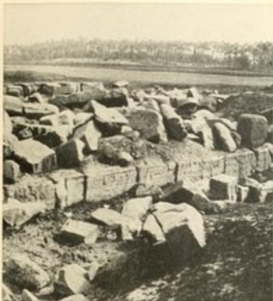
MAIN DOOR WAY.
