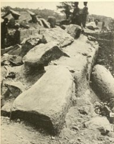
GRANITE DWARF WALL OF ENTRANCE.
