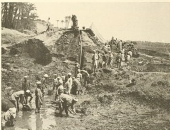
PUMPING OUT THE POND.
