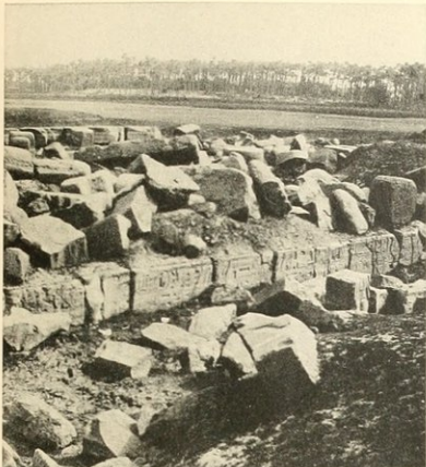
MAIN DOOR WAY.
