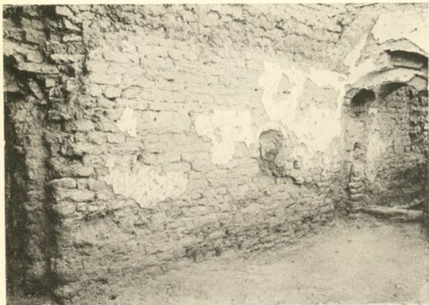
The Castle: Niche and doorways in room 14.
