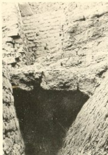
The Castle: Room 11a, showing the method of floor-laying above the vault.
