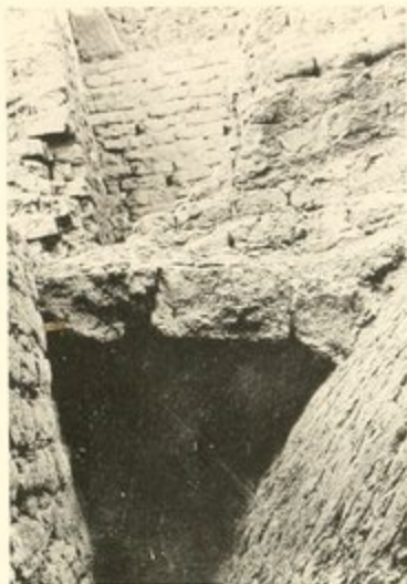
See p. 12 The Castle: Room 11a, showing the method of floor-laying above the vault.
