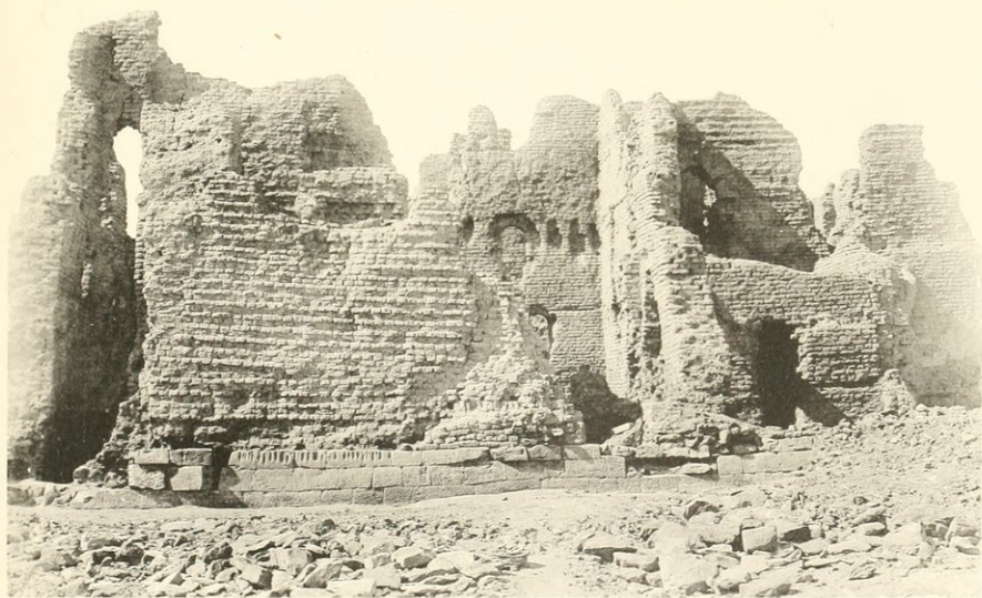
The Castle: The east face showing the repaired gateway.
