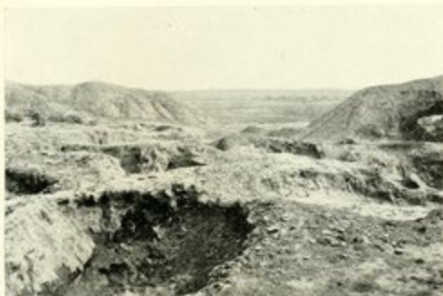
3. N.E. GATE FROM INSIDE.
