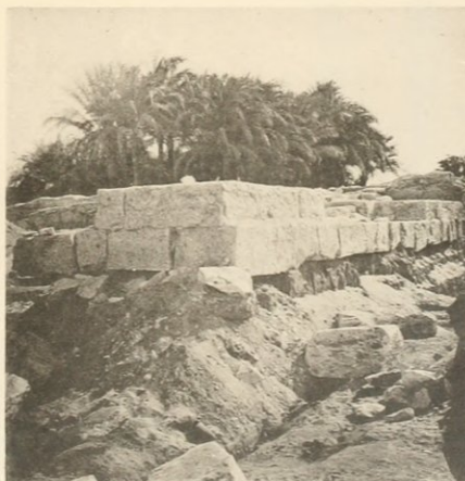
6. FOUNDATIONS OF AAHMES II.
