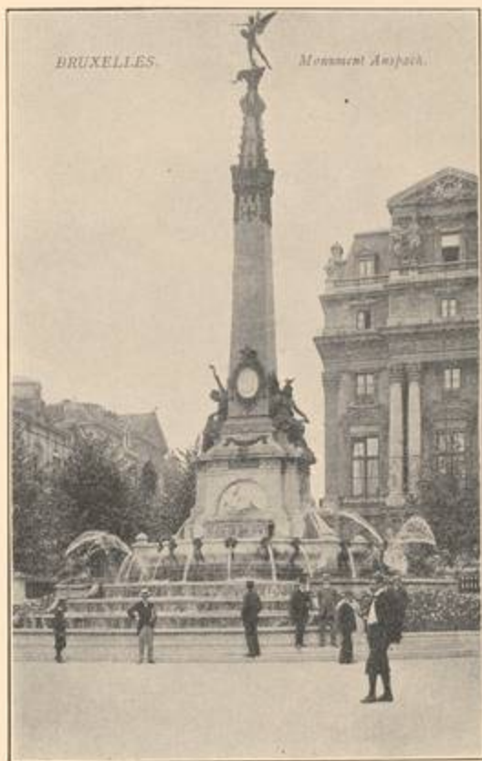
Shaft of Anspach, Brussels, Belgium
