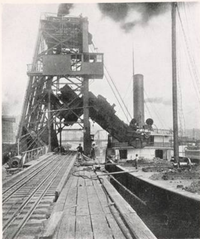
CAR DUMPER IN THE ACT OF TIPPING TRUCK.
