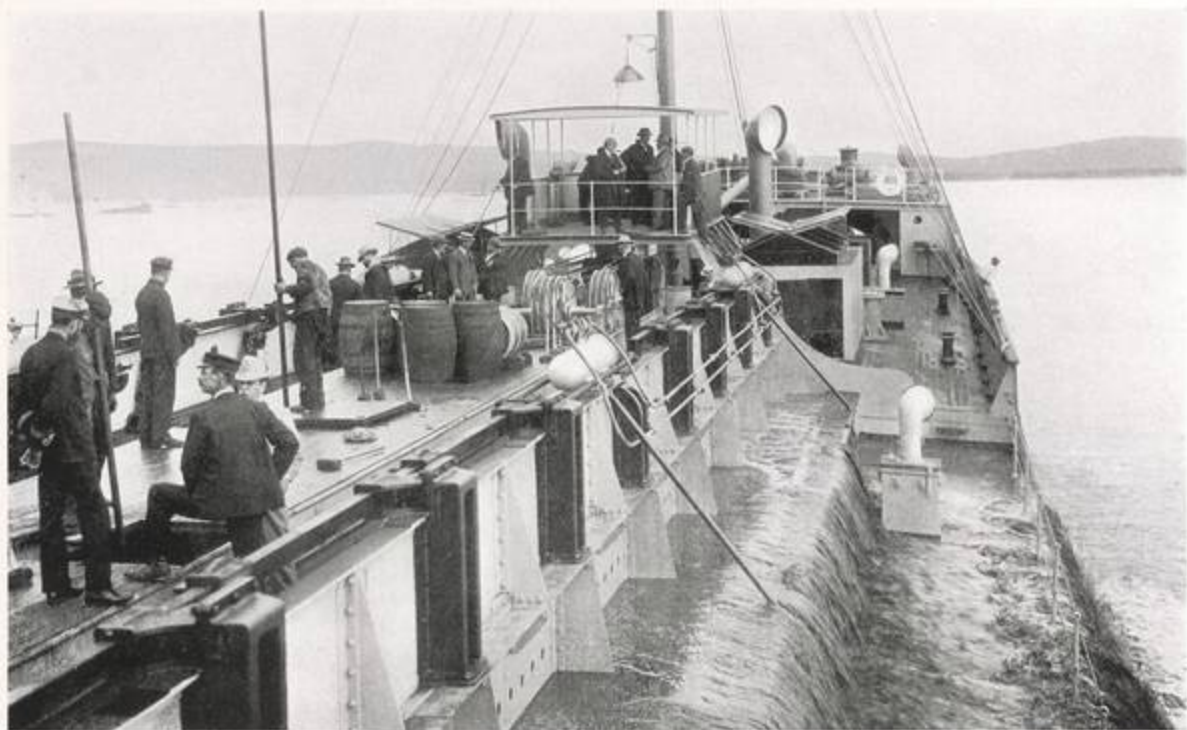
DREDGER "NAUTILUS" (HOPPER CAPACITY, 2,500 TONS) AT WORK IN DURBAN HARBOUR
