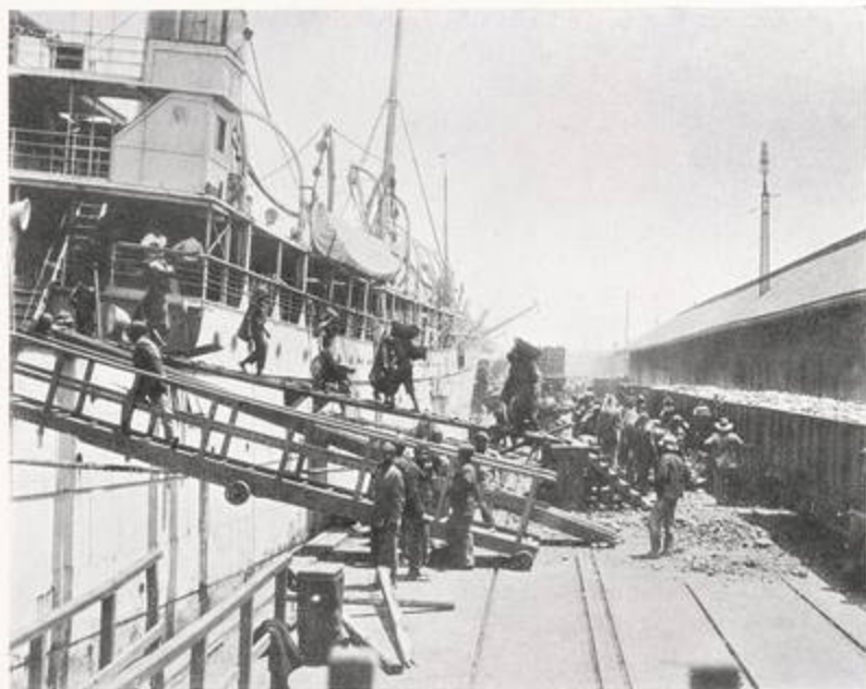
COALING A LINER (THIS METHOD WILL SHORTLY BE SUPERSEDED BY MACHINE APPLIANCES AS SHOWN ON PAGE 6)
