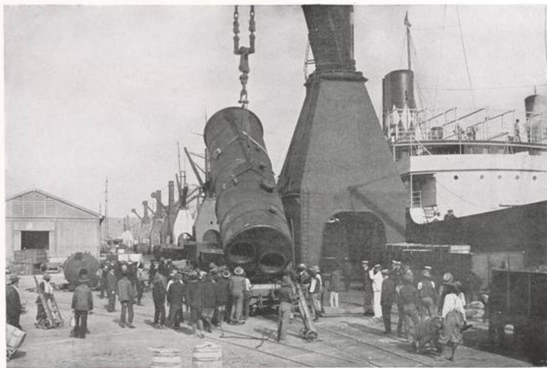
GIANT CRANE LOWERING 25 TON BOILER
