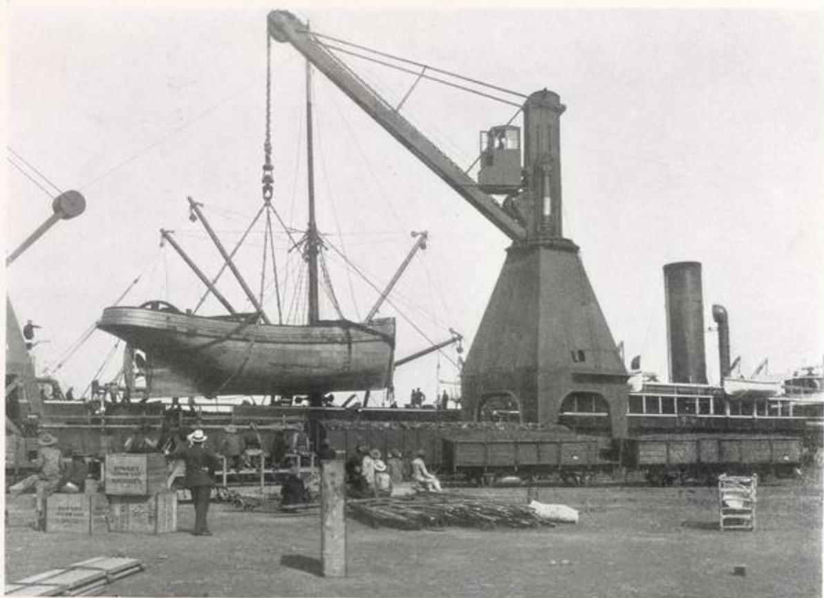
50-TON HYDRAULIC CRANE NEGOTIATING 45-TON LIFT
