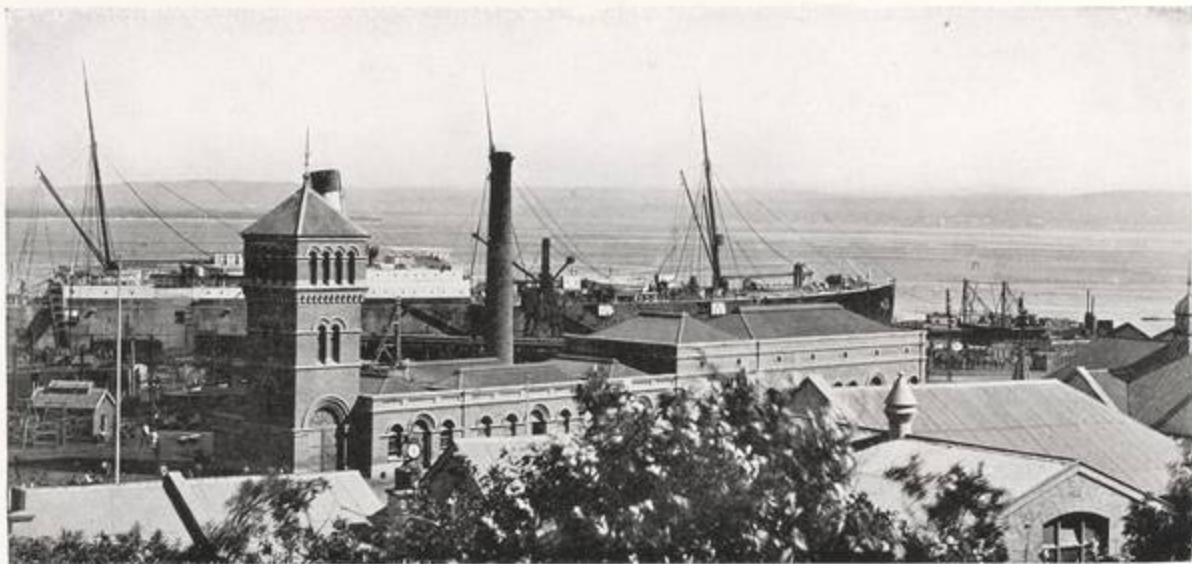
ELECTRIC LIGHT STATION
