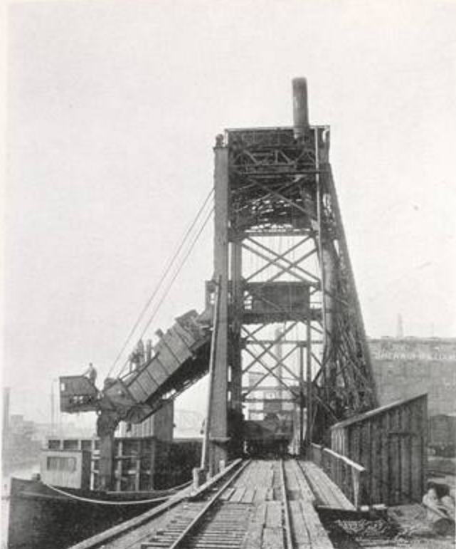
CAR DUMPER, SHOWING TRUCK ON CRADLE READY FOR HOISTING.
