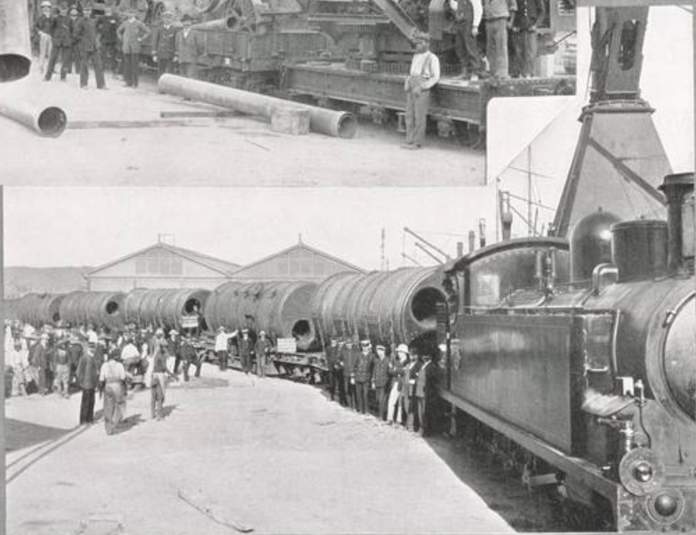
TRAIN OF BOILERS. WIDTH 10\frac{1}{2} FEET. EACH WEIGHING 25 TONS, LENGTH 33 FEET
