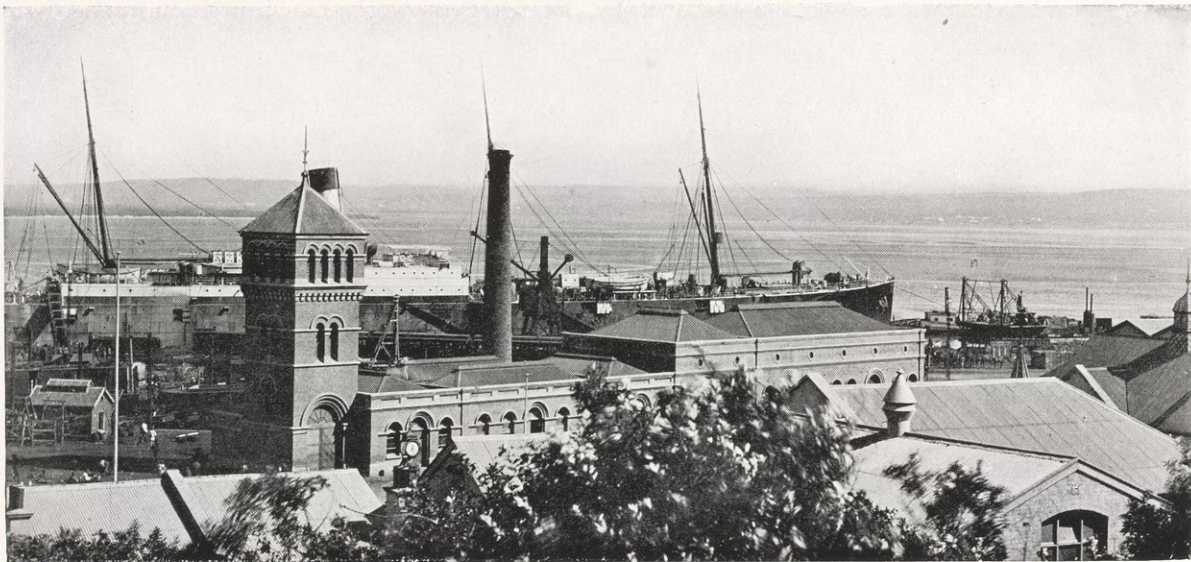
ELECTRIC LIGHT STATION
