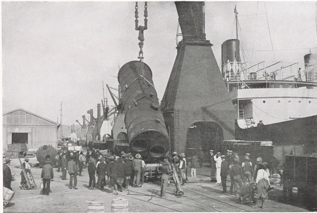
GIANT CRANE LOWERING 25 TON BOILER
