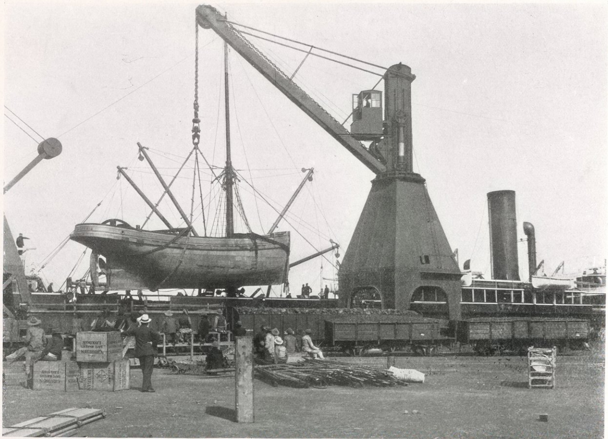
50-TON HYDRAULIC CRANE NEGOTIATING 45-TON LIFT
