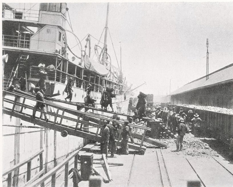
COALING A LINER (THIS METHOD WILL SHORTLY BE SUPERSEDED BY MACHINE APPLIANCES AS SHOWN ON PAGE 6)
