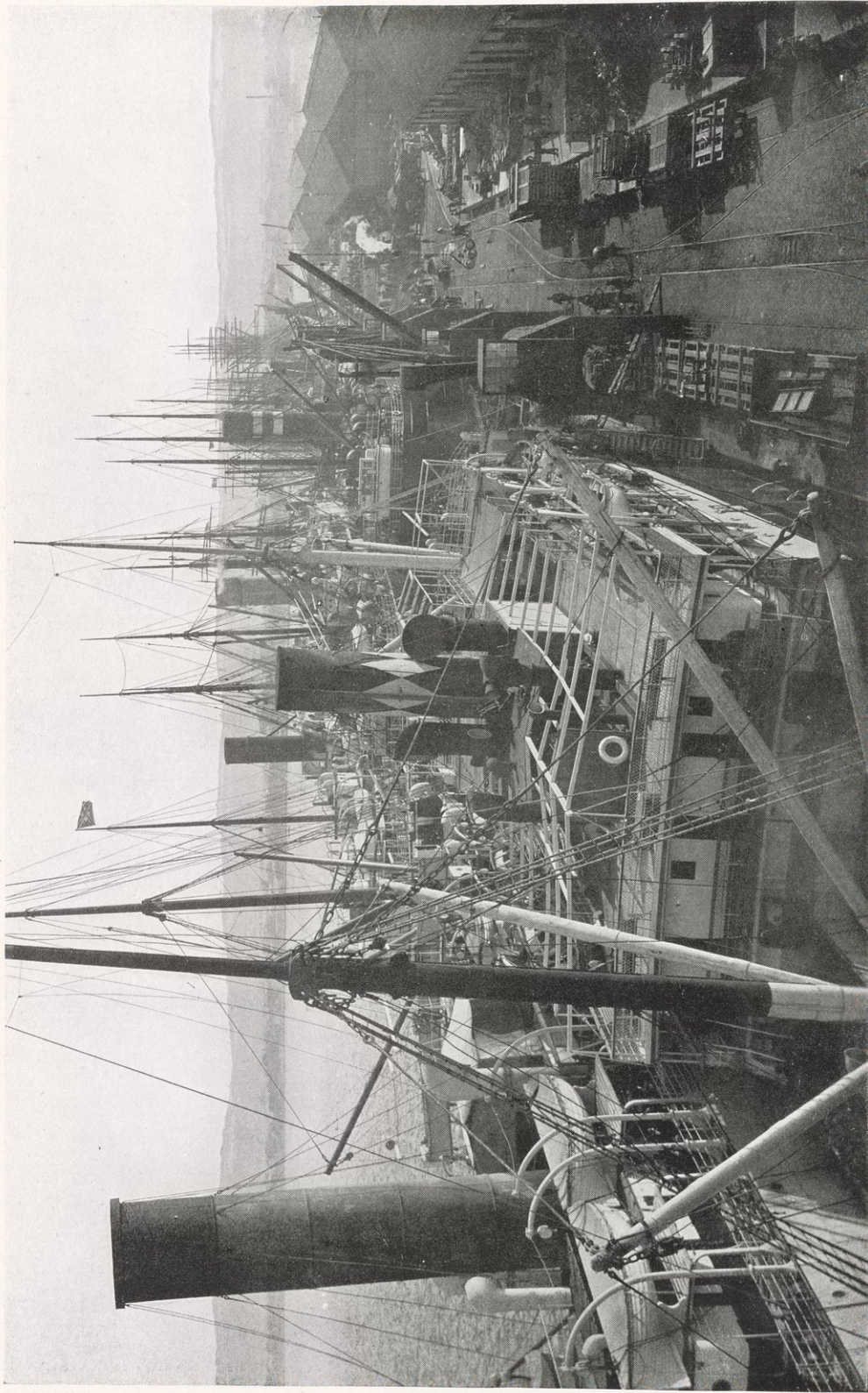
BERTHAGE AND WHARFAGE—PORT NATAL View taken on 30th June, 1902, showing a portion of the Permanent Wharfage, Sheds, Hydraulic Cranes, and Berthage towards of the 50-ton Crane, together with an aggregate of 47,709 tons of Shipping lying alongside, viz.: 6 Steamers, 38,955 tons, and 9 Sailers, 8,754 tons. Five years previous to date of photograph, this spot was a sandbank dry at Low Water.
