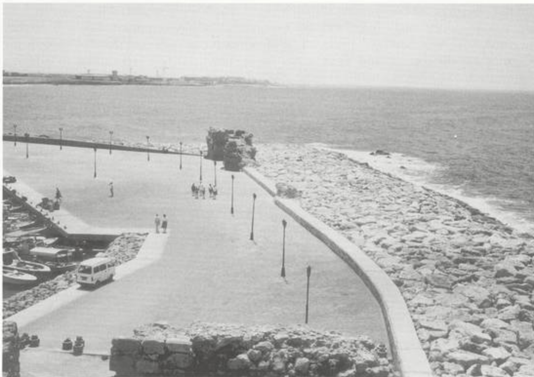
Figure 8. Renovations to the western breakwater at Paphos in the 1980s, namely, the addition of a ca. 23 m. wide rubble baffle, allowed the port authorities to remove a seawall that had once formed the main defensive line against storms. Ruins in the sea south of the remains of the Frankish Fort mark the line of the ancient spur. Photograph by R. L. Hohlfelder (looking E)
