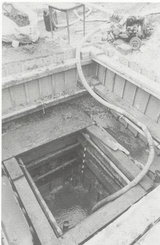
Figure 30. The shored probe (locus 700) in I14. Photograph by Zaraza Friedman
