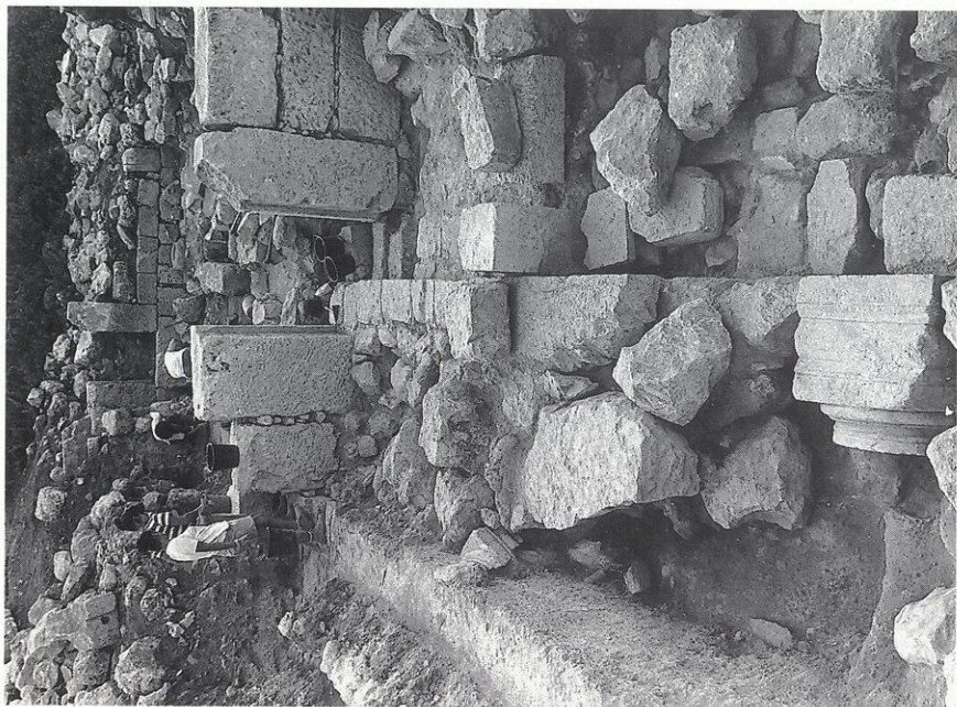
8b. H. Sumaqa: (W2 in L291). The wall is composed of a hard mixture of stones and concrete and makes use of many architectural fragments. View is from west to east.
