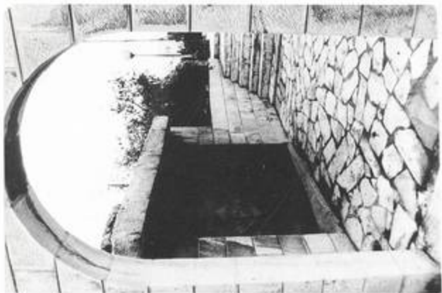
Fig. 4.7 'Amman Citadel—access to the underground water reservoir
