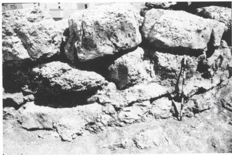
Fig. 4.10 The plaster on the exterior face of the tower at Khilda
