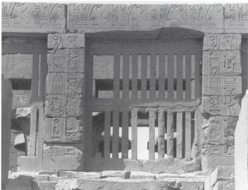
98. View of the south exterior face of the clerestory of the Karnak Hypostyle Hall.
