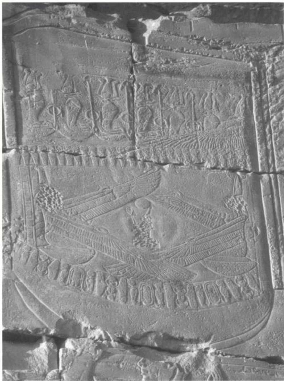
148. Canopy of Amen's barque with rebus of Tutankhamen usurped by Seti I, Karnak Eighth Pylon, north face. Key Plans KG 104 .
