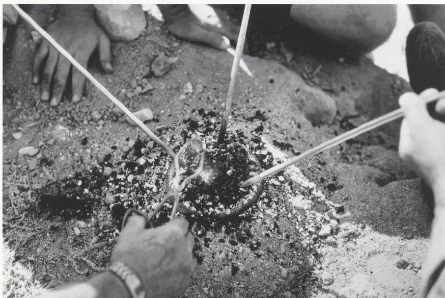
Plate 17: Experimental Smelt, Celaller Village using three blowpipes.
